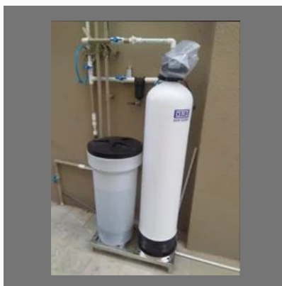
Org Automatic Water Softener
